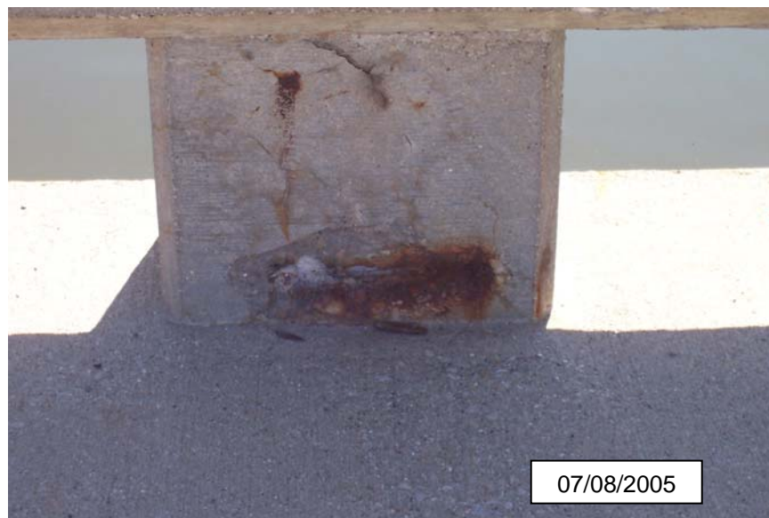
Photograph 22 - Representative parapet base spalling
