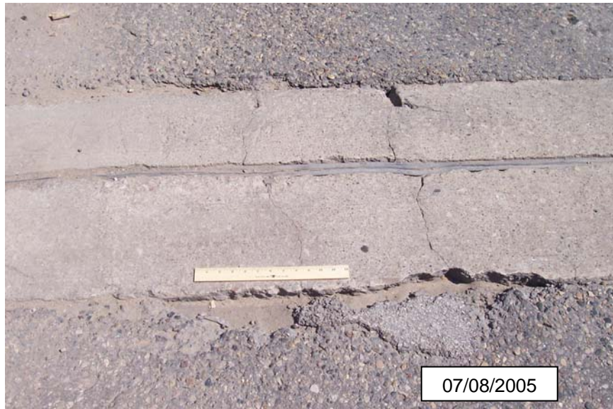
Photograph 24 - Asphalt condition at Pier 1 Expansion Joint
