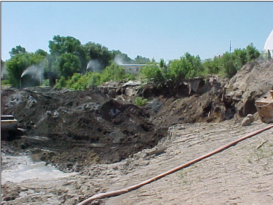
PHOTO 8—Water misters operating downwind of the work area in June 2006.
