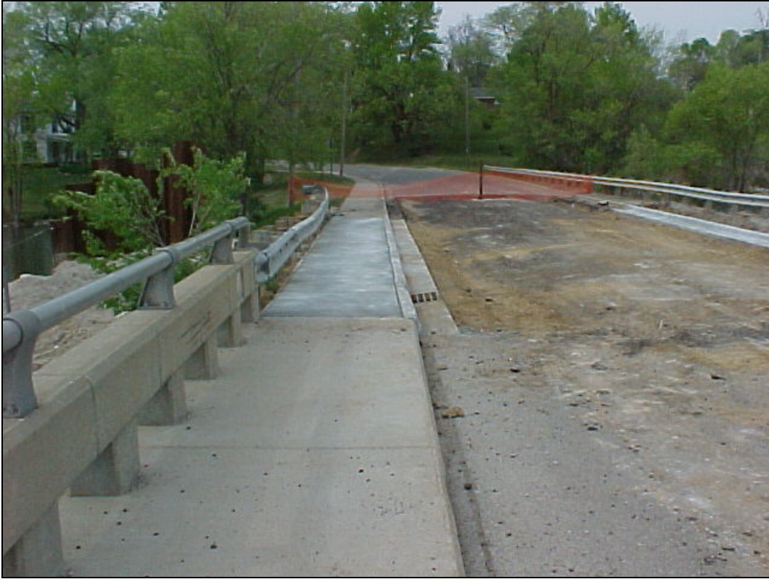
PHOTO 7—Previously damaged sidewalk after replacement in May 2006.
