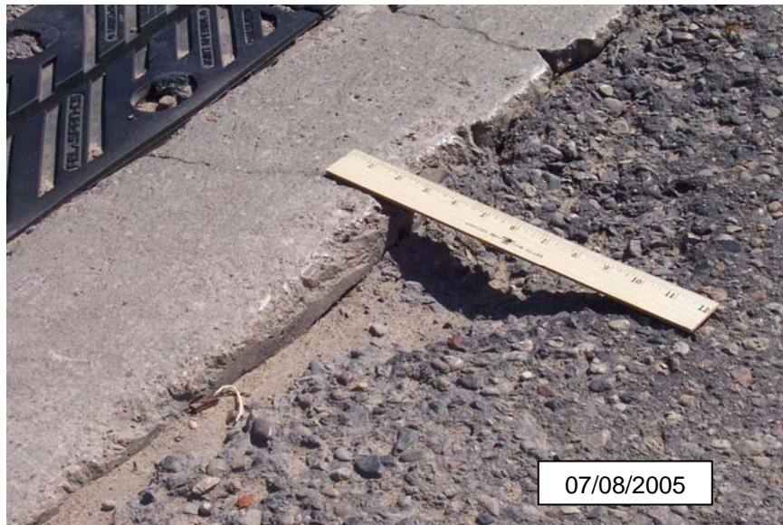
Photograph 23 - Asphalt condition at Pier 2 Expansion Joint
