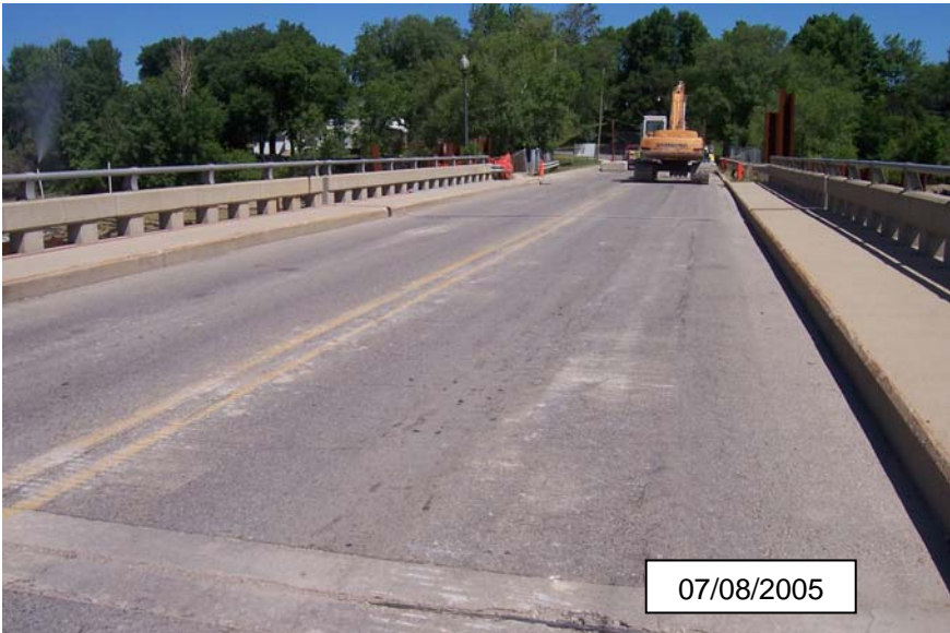
Photograph 2 - Looking North along structure
