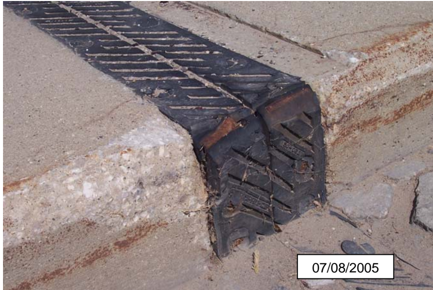
Photograph 25 - Pier 2 expansion joint damage
