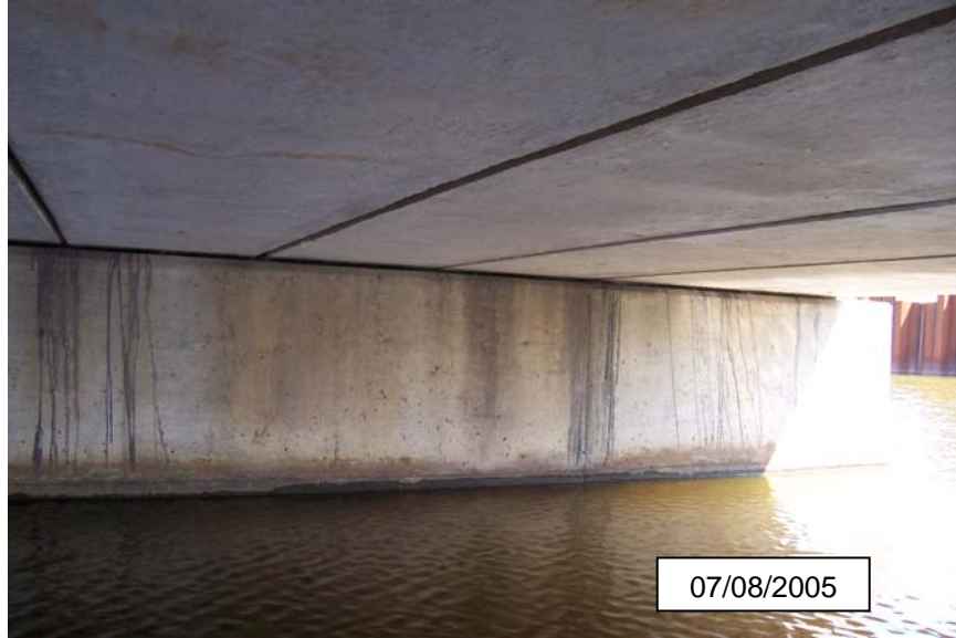
Photograph 17 - Beams at Span 1
