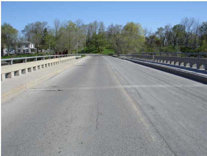
Photograph 2 - Looking North along structure
