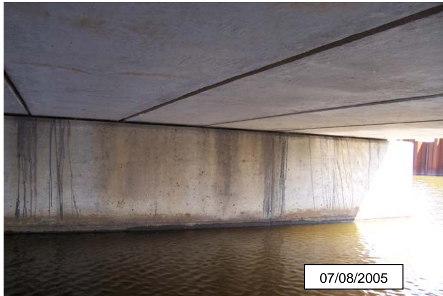
Photograph 16 - South face of Pier 1
