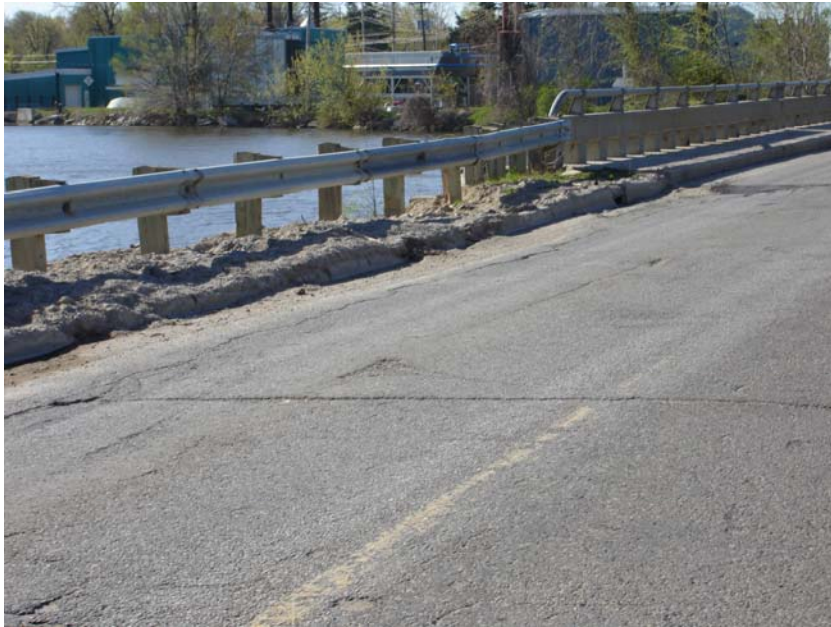
Photograph 5 - Northeast curb and guardrail removed
