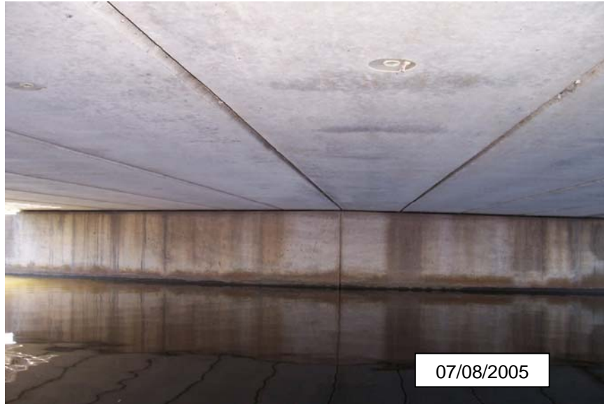
Photograph 15 - North face of Pier 1
